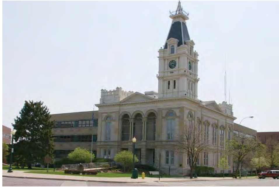
Monroe County Courthouse
