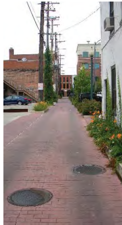
Storm and Sanitary Access in Downtown Monroe
